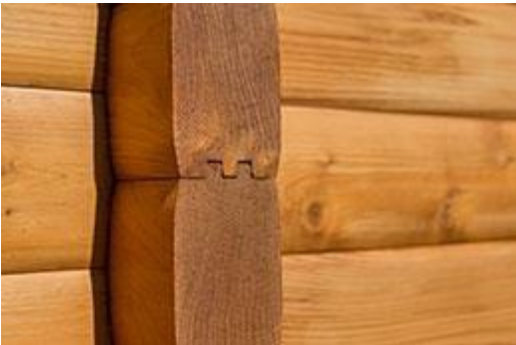
Figure 4-18. Timber Frame House Joins
