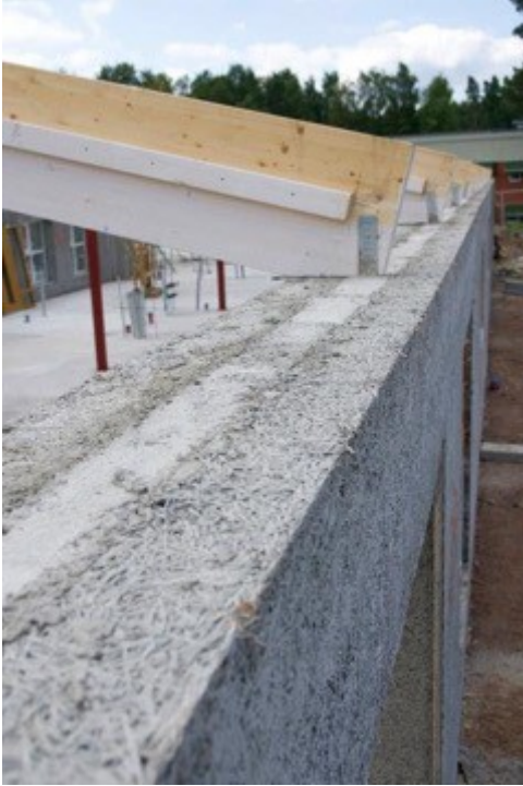
Figure 4-14. Wood Wool Cement Building Application
