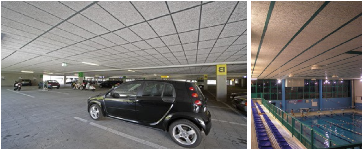
Figure 4-12. Wood Wool Cement Applications
