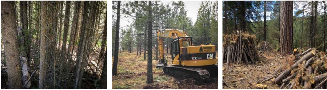
Figure 2-5. Sagehen Creek Experimental Forest Mechanical Treatments and Slash Piles, 2017, Faerthen Felix
